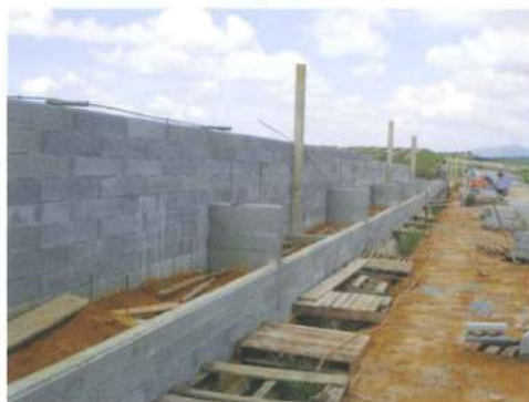
Retaining Wall - Planter Box
