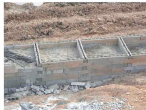
Retaining Wall - Foundation Box
